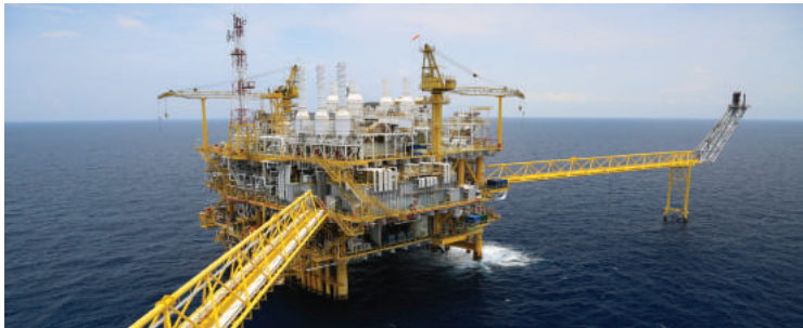
Major Supply ; "Gumusut Kakap FPS", "BP Angola FPSO PSVM", "FPSO Kwame Nkrumah".
